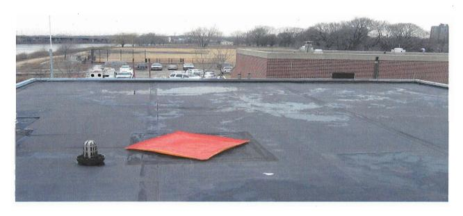
Rooftop Drain where Fuel Oil Leaked through Internal Piping to Charles River
