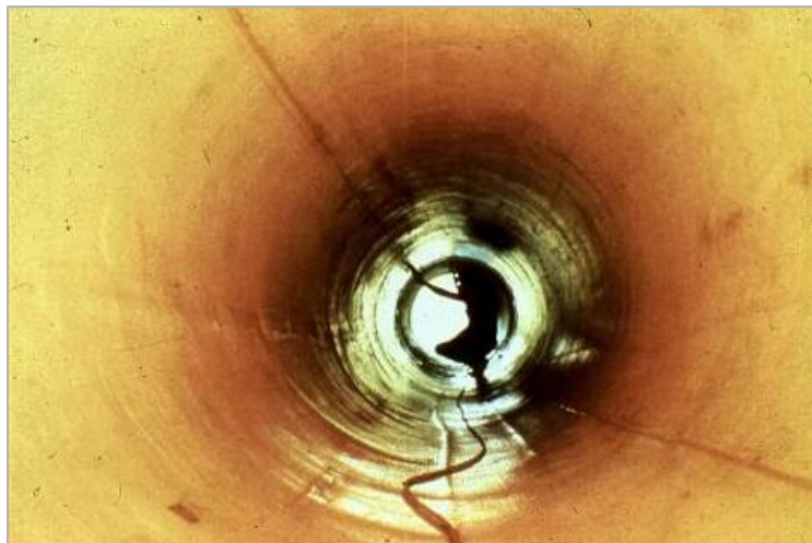
Example of sewer rehabilitated with cured-in-place liner
