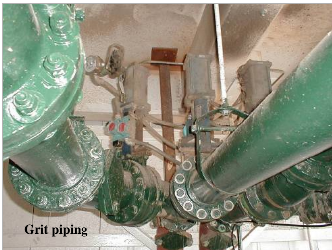
Photos above show grit piping and grit collection pod typical of all three older remote headworks – Chelsea Creek, Columbus Park and Ward Street. The grit removal systems are in need of replacement.
