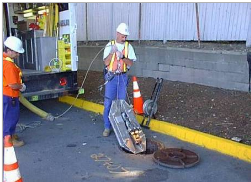
TV Inspection Crew
