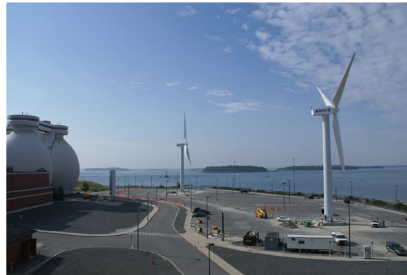
Wind Turbines at Deer Island, next to Anaerobic Gas Digesters
