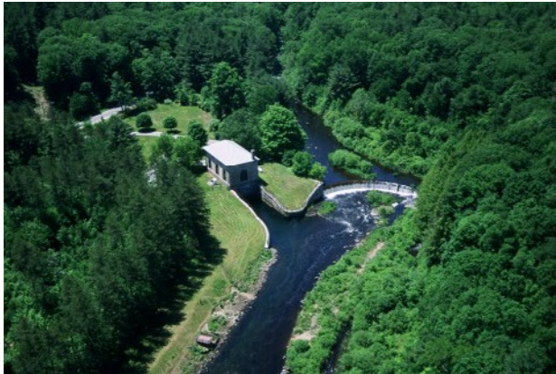
The Oakdale Hydroelectric Generation facility captures energy as water enters the Wachusett Reservoir from the Quabbin Reservoir.
