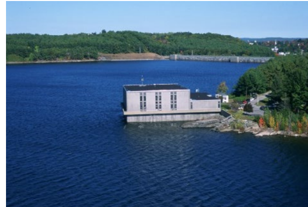
Hydroelectric generators at the Cosgrove Intake capture energy as water leaves the Wachusett Reservoir headed toward metropolitan Boston area.
