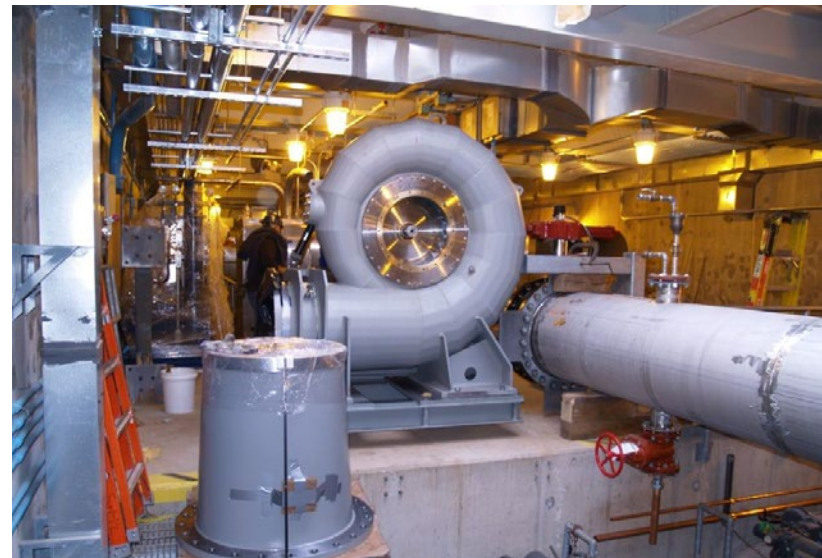
Loring Road Hydroelectric Generator during construction
