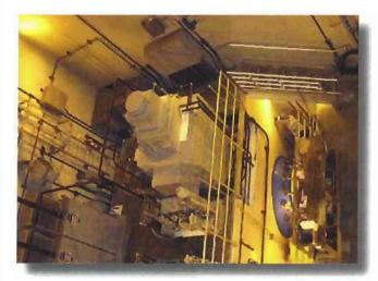
Since 2002, energy is recovered at Deer Island by the flow of treated wastewater as it drops from the plant into the outfall tunnel shaft through two one-megawatt hydroelectric generators that produce over 5 million kW hours per year and provide an annual savings in electrical costs of \$600,000.
