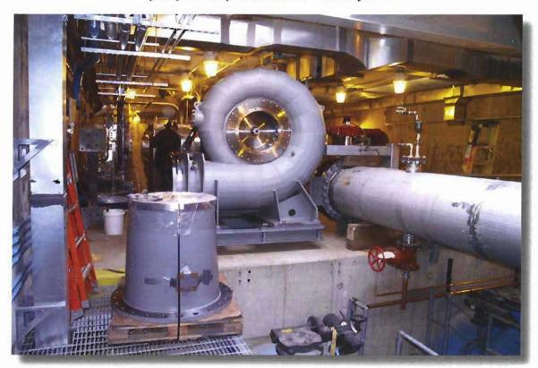
In Weston, a new hydroelectric generator has been installed at the Loring Road covered storage facility, which will generate 1.2 million kilowatt hours per year. This \$1.8 million project is fully funded through ARRA and the Massachusetts Technology Collaborative and will provide an annual savings in electrical costs of \$150,000.
