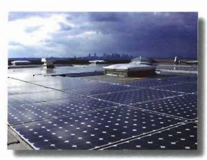
A 180-kW roof-mounted solar photovoltaic system was installed on the Administration/Warehouse roof in fall 2009. This \$1.2 million design/build project was partially funded through ARRA and provides an annual savings in electrical costs of \$19,000.
