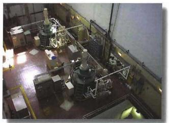
MWRA also operates hydroelectric generators where the drinking water enters and leaves the Wachusett Reservoir. At Oakdale, a 3.5 MW turbine generates 13 million kilowatt hours per year and at Cosgrove, two 1.7 MW turbines generate 3 million kilowatt hours per year and provide an annual revenue from efectrical sales of \$1.1 million.
