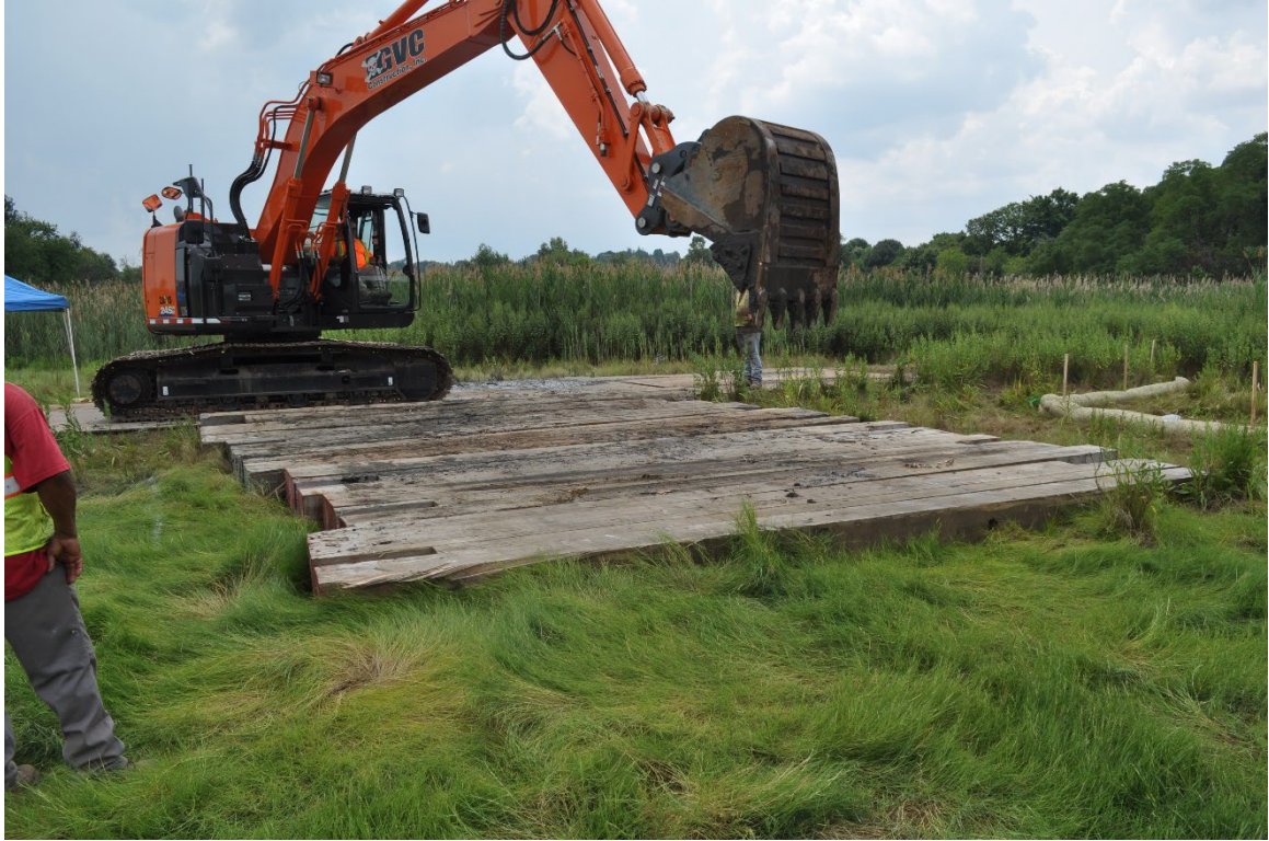
Photo 3-1 Timber Mats Being Placed for 2020 Test Pit
