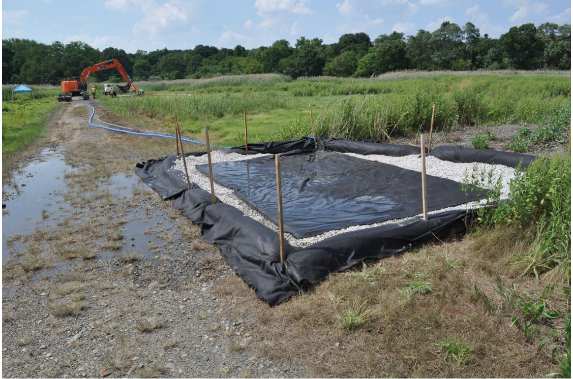
Photo 3-4 Dewatering Filter Basin During 2020 Test Pit
