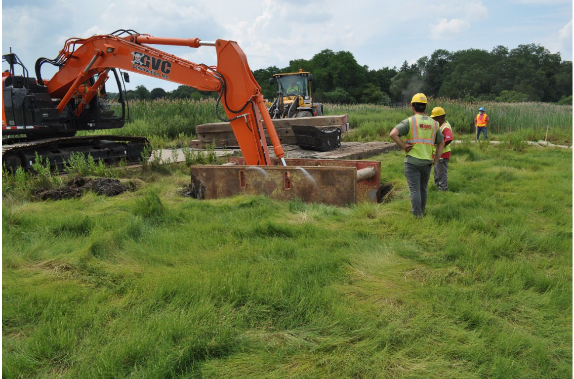
Photo 3-3 Trench Box Support of Excavation Being Placed During 2020 Test Pit
