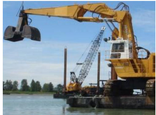
Figure 43 - Clamshell Bucket on Excavator
