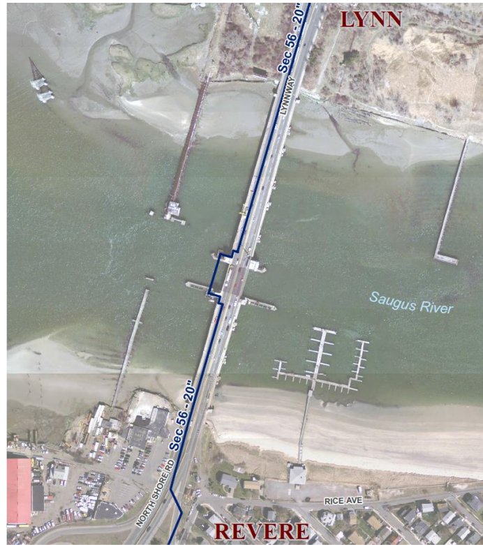
Figure 3- Orthophoto of General Edwards Bridge
