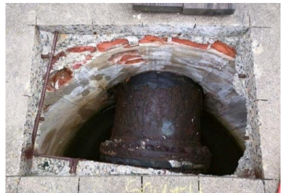
Figure 12 - Inside South Tunnel Shaft
