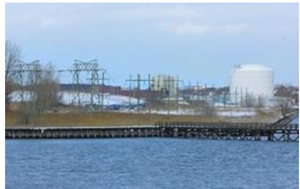
Figure 19 - Historic Power Lines in Harbor Area
