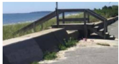
Figure 24 - Revere Seawall (East)
