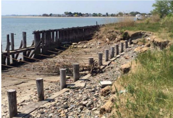
Figure 25 - Lynn Seawall (East)
