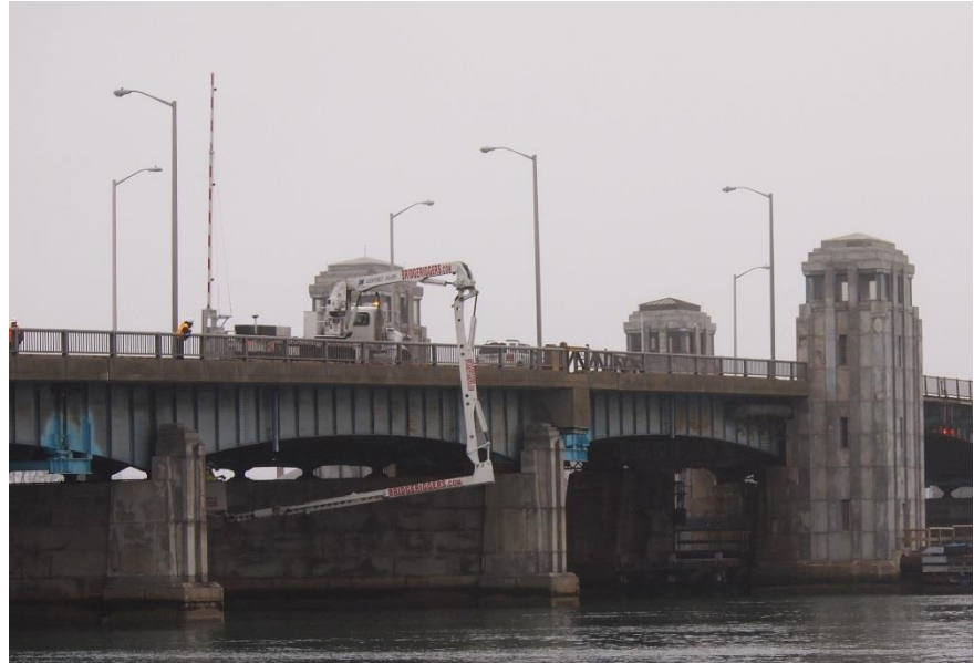
Figure 16 - Accessing Section 56 via Snooper Truck
