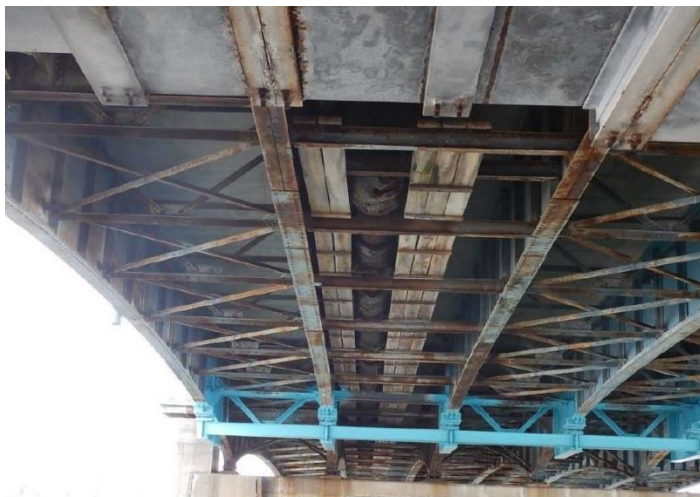
Figure 4 - Typical Configuration of Pipe, Support Beams, and Timber Plank Walkway
