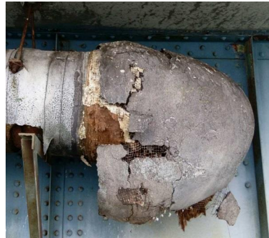
Figure 15 - Fibrous Insulation Sample Location No 4
