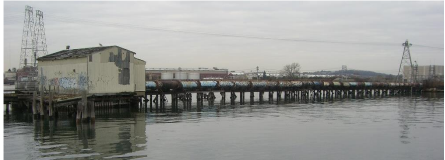
Figure 18 - Historic Railroad Bridge (North)
