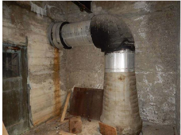
Figure 10 - South Tower Pipe Condition
