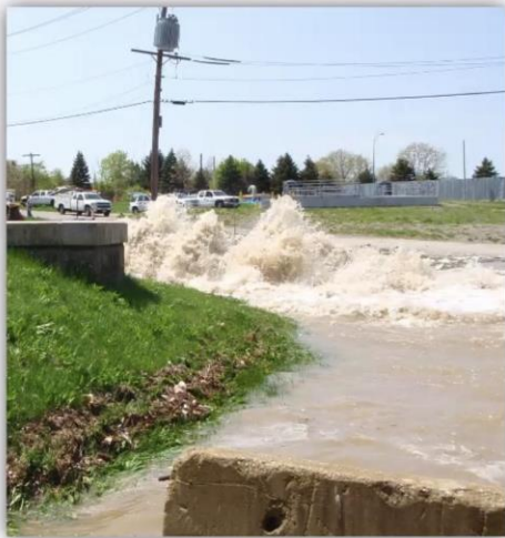
250 MGD flow at Shaft 5 break....
