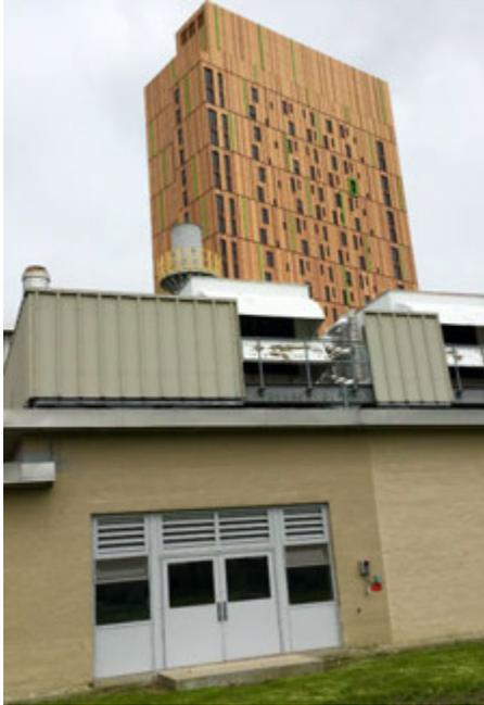
← To the left, the exhaust stacks at Ward. On the left is the boiler stack. A generator stack is to the far left. MassArt's dormitory is behind.
