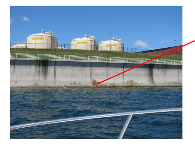
Concrete deterioration and exposed reinforcing steel
