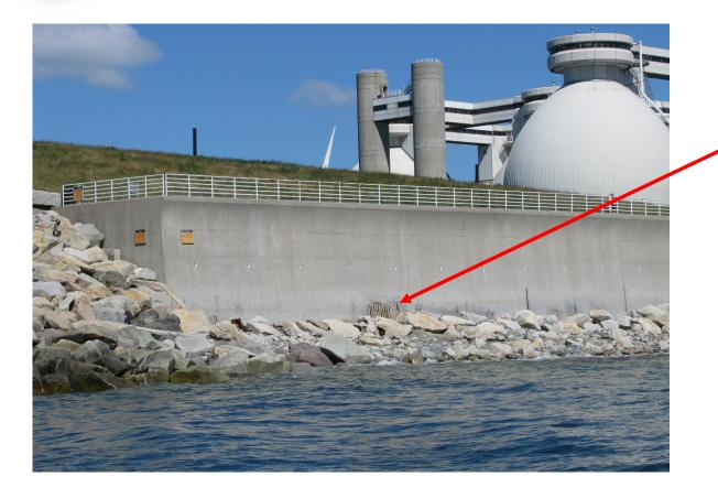
Concrete deterioration and exposed reinforcing steel
