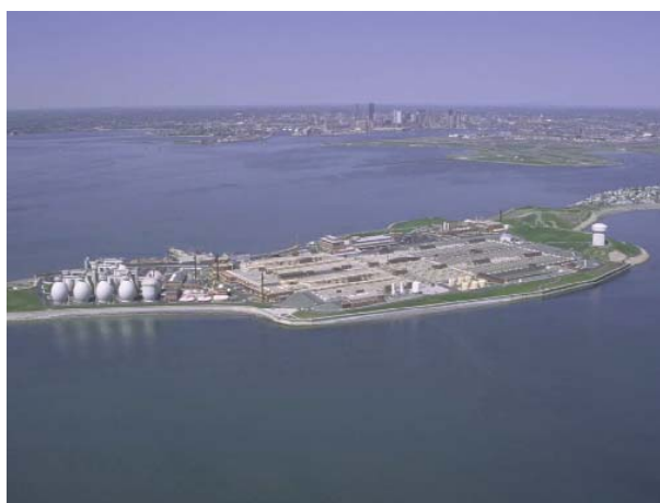
Fig. 1. Deer Island wastewater treatment facility with City of Boston in background.
