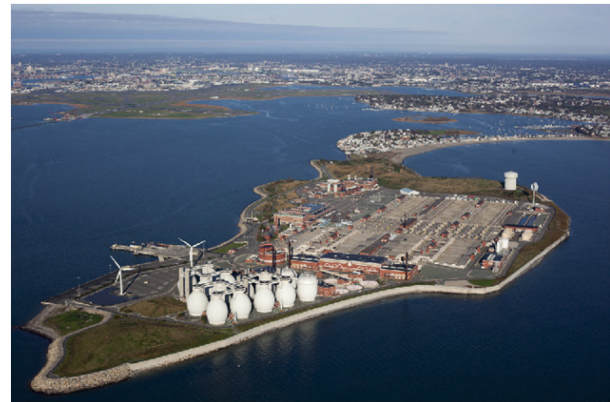
Fig. 1. Deer Island wastewater treatment facility with City of Boston in background.
