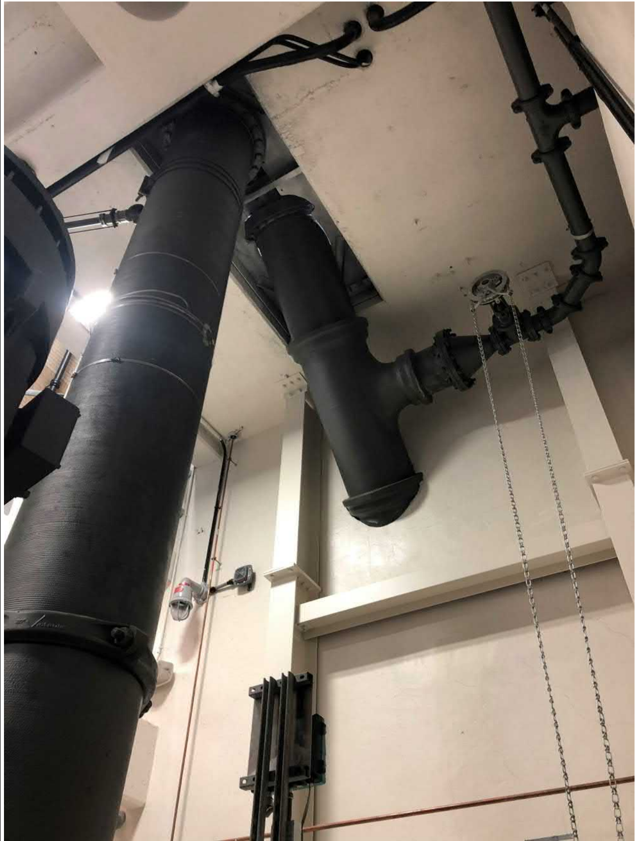
Figure B.3: Dry weather pump discharge piping
