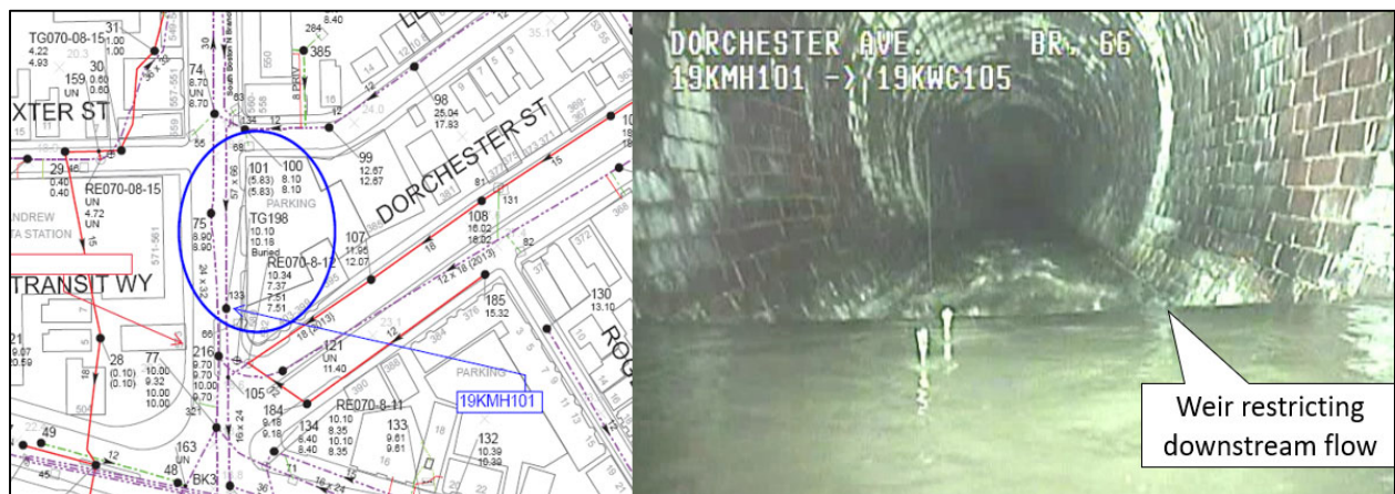
Figure 5-2. Weir Restriction on Dorchester Ave.
