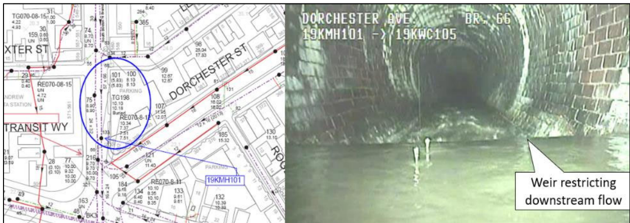
Figure 5-2. Weir Restriction on Dorchester Ave.
