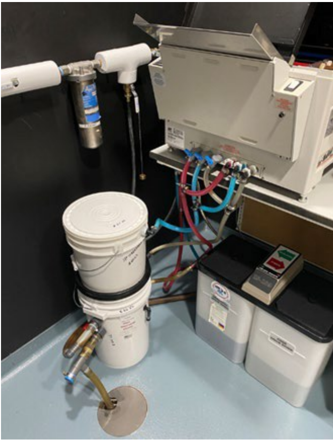
Figure 1: SIU inspection of silver recovery unit
