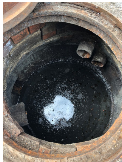
Figure 2. Inspection of an existing gas/oil separator.
