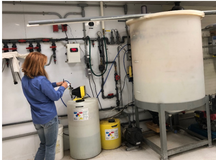
Figure 1. Inspection of treatment system at an industry.
