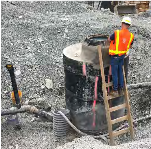
Figure 2. Inspection of a new gas/oil separator.
