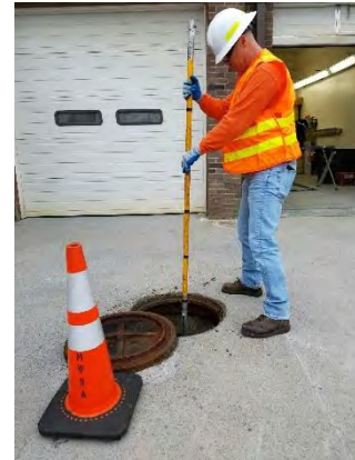
Figure 2. Inspection of a gas/oil separator.
