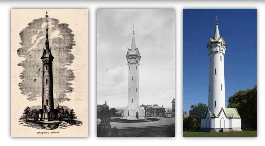
• The standpipe was a 5-foot diameter iron plate tank inside a masonry structure, it took over the role of supplying Beacon Hill and Dorchester Heights, as well as supplying Roxbury Heights
