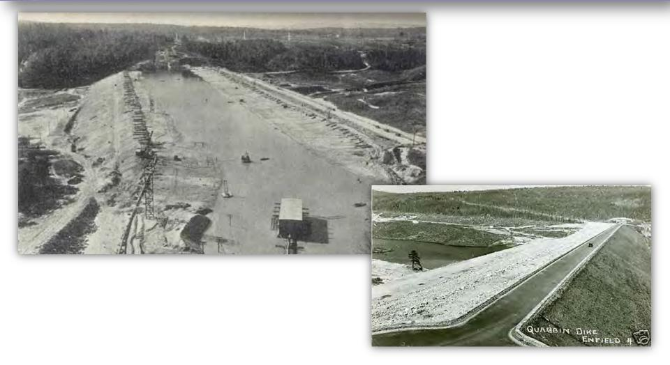
Soil for the earth dam was quarried and mixed with water to make a slurry, then pumped up and discharged from pipelines along the edge of the rising dam. The water would seep away and the soil would build up the dam.
