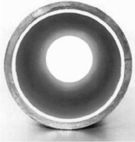
WATER PIPE AFTER CLEANING AND LINING.
