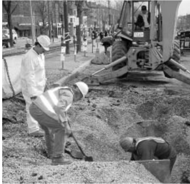
CONTRACTOR PREPARING ONE OF THE ACCESS PITS ON BEACON STREET.
