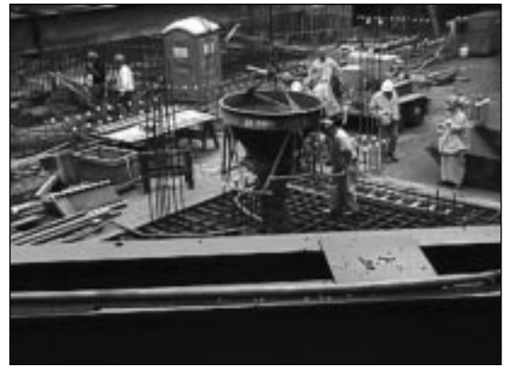
On a similar project, workers prepare for a below-grade concrete pour.
